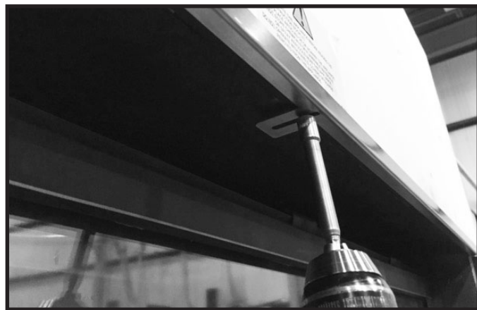
Figure 10.5 Install Trim Ring
