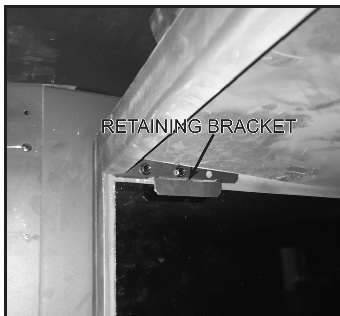
Figure 5 Retaining Bracket Installation - Side Panel
