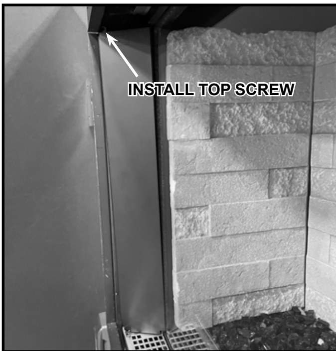
Figure 4.11 Transition Panel installed
