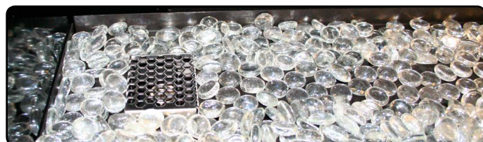
Figure 24.b Completed firestone installation
