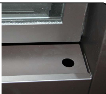
Figure 23.b Removing and installing the Horizontal Access Panel
