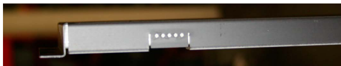
Figure 4.c Bottom of Nailing Flange Extension
