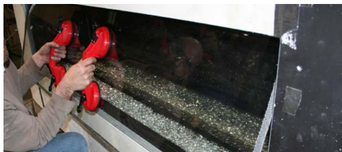
Figure 11.c Window Removal (using glass lifting tools).
