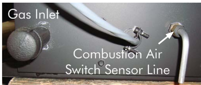
Figure 9.b.b Identifying the Gas Inlet and Combustion Air Switch Sensor Line
