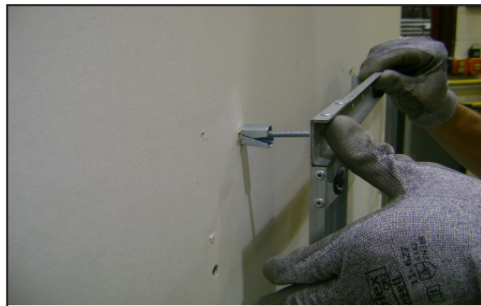
Figure 4.6 Installing Anchors in Hollow Wall
