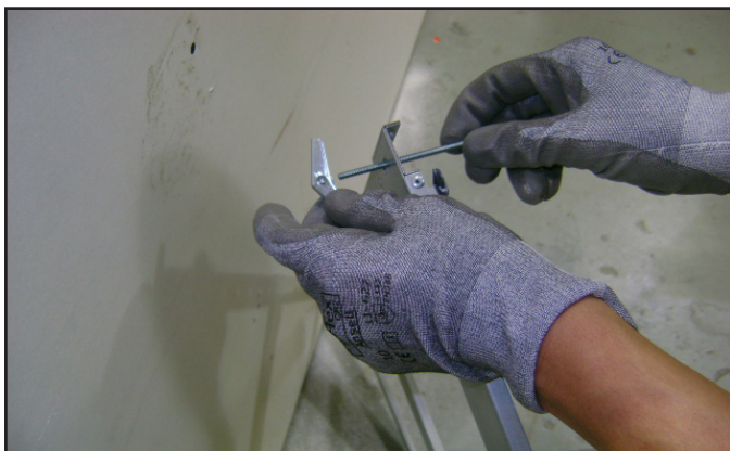
Figure 4.5 Toggle Bolt Installation through Mounting Bracket
